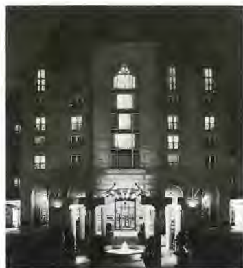
In The Hotel Crescent Court
